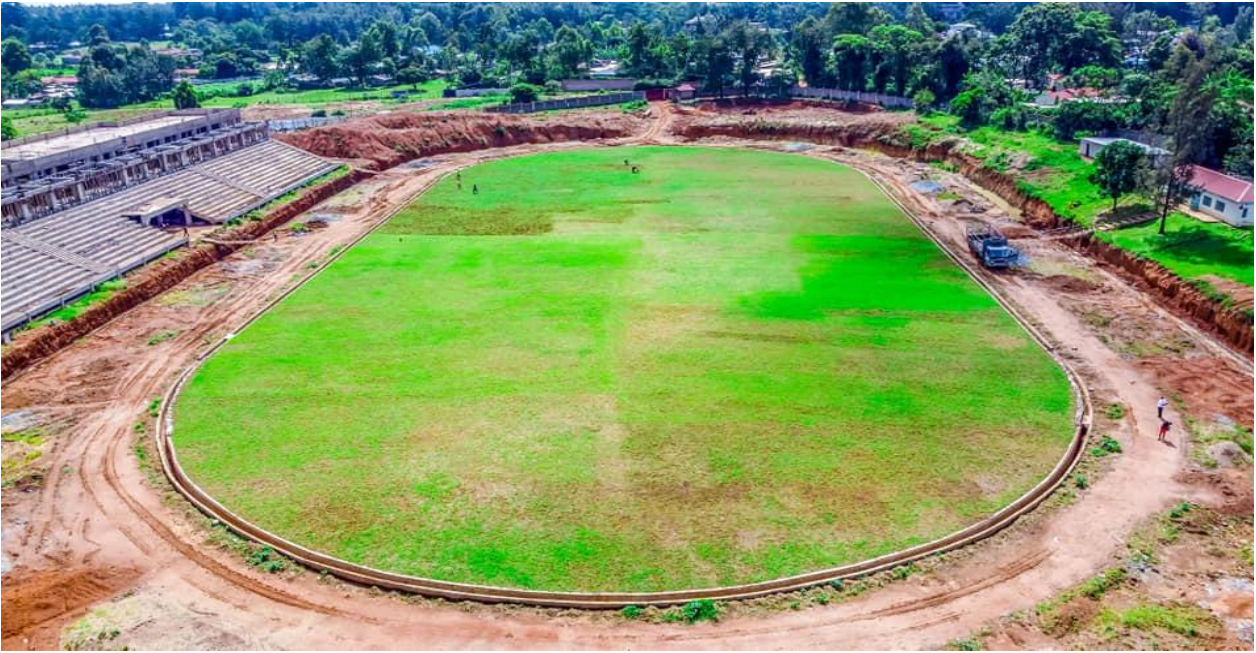
Upgrading of Masinde Muliro stadium in Kanduyi
